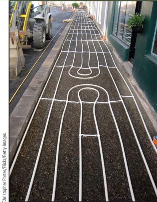
Figure 15.7: Construction of a sidewalk in Reykjavik, Iceland, utilizing heating pipes carrying geothermally heated water to prevent icing.
