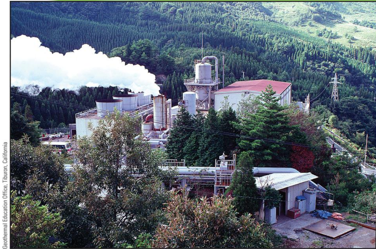
Figure 15.12: Flash steam geothermal power plant in Otake, Japan.
